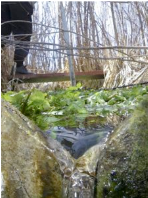
The photo on the left shows the “V” notch of the weir with the clear spring water topped with watercress. On the right you can see the water dropping down to the level of the Rio Bonito.
