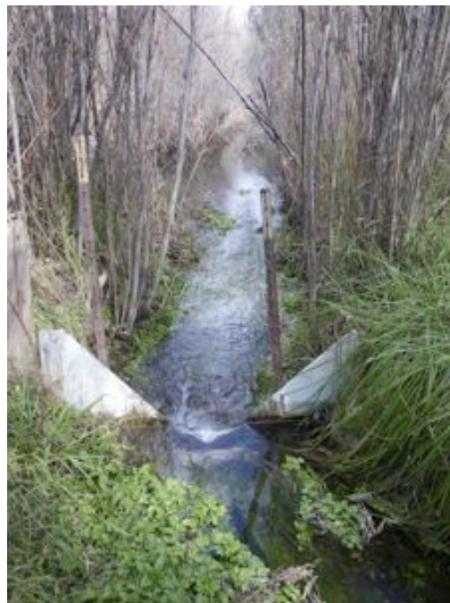
The photo on the left shows the “V” notch of the weir with the clear spring water topped with watercress. On the right you can see the water dropping down to the level of the Rio Bonito.
